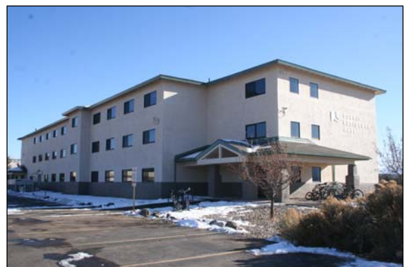
CMC Glenwood Springs Dormitory
